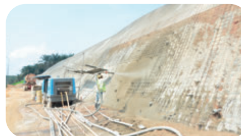
Soil nailing works and guniting (spraying of dry concrete mixture) works are being carried out to improve and stabilise the slopes
