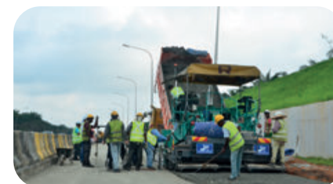
Laying of CBM 4 layer for pavement at the New Slow Lane
